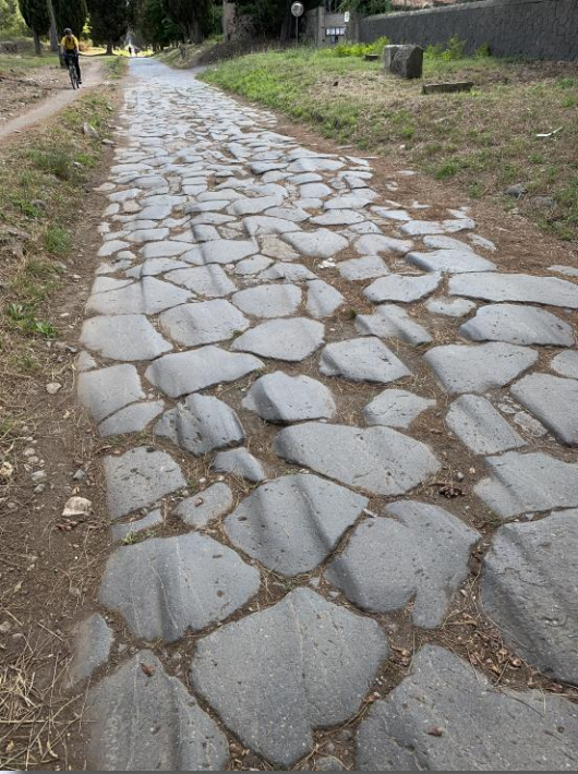
Top: This is what real cart ruts look like on the Via Appia in Rome. Keep in mind that wheels from ox and horse carts in Roman times already had metal rims, that wore down the rock faster than plain wooden wheels. Source: Wikipedia
